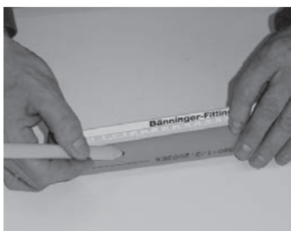
Fig. 5 Mark out the socket depth.
